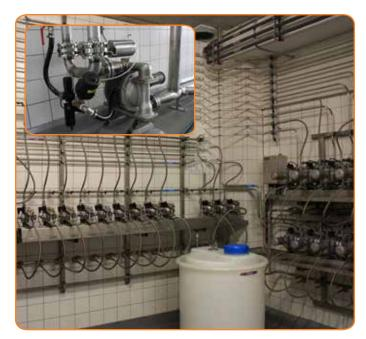
Chemical usage is one of the main cost considerations in a tank-cleaning operation and Wilden® AODD pumps offer the leak-free operation and accurate dosing that helps optimize that chemical usage.
