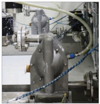
Villeroy & Boch utilizes three Almatec<sup>®</sup> CHEMICOR Series AODD Pumps to transfer various oils and color pastes at its Wellness plant.
