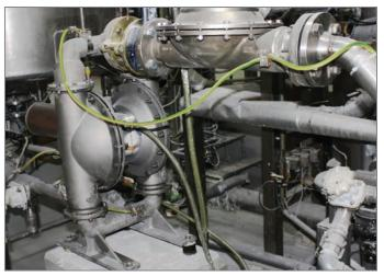
Reliability is a key characteristic of the Wilden<sup>®</sup> Advanced<sup>®</sup> Series AODD Pumps as a single pump is required to pump base polymers to 11 different machines around the clock in Villeroy & Boch's Wellness manufacturing operation.
