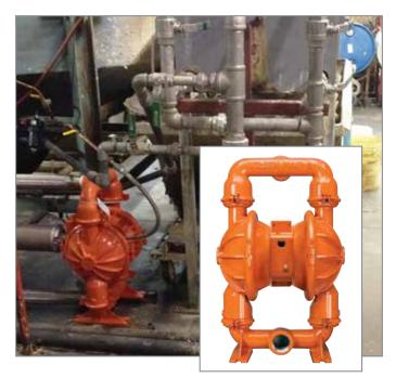
Wilden® AODD pumps with Pro-Flo® SHIFT™ Air Distribution Systems meet the heavy demands of forcing waste-laden sludge into the filter press chambers for water/ waste separation. AMTROL utilizes Wilden AODD pumps exclusively for all fluid-transfer applications at its manufacturing facilities because of their proven effectiveness in a variety of demanding applications.
