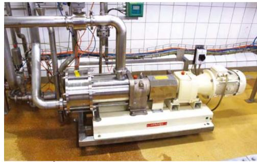
What sets the Mouvex® SLS Series Eccentric Disc Pump apart is an innovative seal-less design that incorporates a hermetic pump head with a self-adjusting eccentric shaft protected by a double-wall stainless-steel bellows that ensure long life and product safety.
