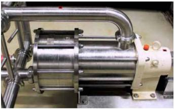
When selecting pumps, wine producers must choose a pumping technology that possesses the ability to recover expensive products and ingredients from the tank and piping systems. This is why Bailly Lapierre chose to install Mouvex® SLS Series Eccentric Disc Pumps.
