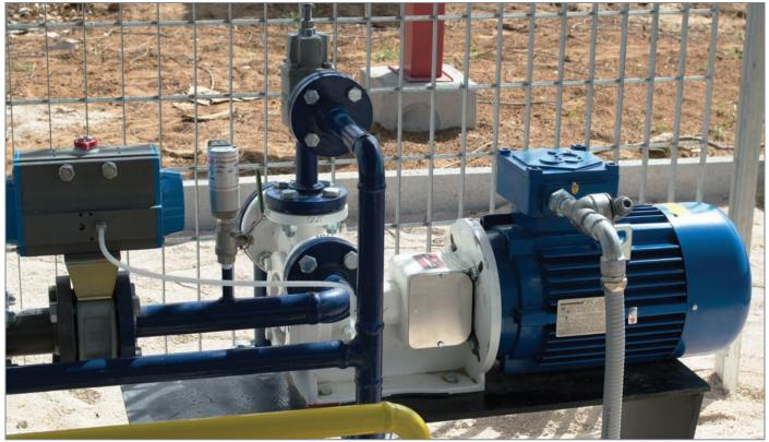
Ebsray® RC40 Series Regenerative Turbine Pumps feature a motor that is smaller than competitive pumps, resulting in energy-cost savings. Despite the smaller motor, the RC40 pump will easily, reliably and economically produce differential pressures up to 14 bar (200 psi) with flow rates up to 200 L/min (52.8 gpm).
