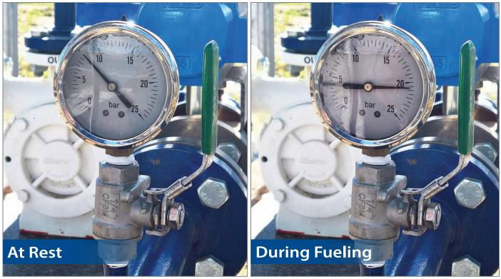
A key to uninterrupted Autogas dispensing in Italy's warm summer months is utilizing a storage-tank pump that can create enough differential pressure between it and the vehicle's fuel tank. At rest, the Autogas storage tank at AmeGas' site in Sabaudia has a pressure of 8 bar (116 psi), left photo, but when fueling begins, the Ebsray® RC40 Series Regenerative Turbine Pump can create 21 bar (305 psi) of pressure, which is more than enough to facilitate the fueling process.
