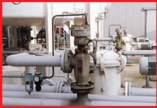
In-Line PFM Systems for modern LOBP operation installed with local control pressure regulator
